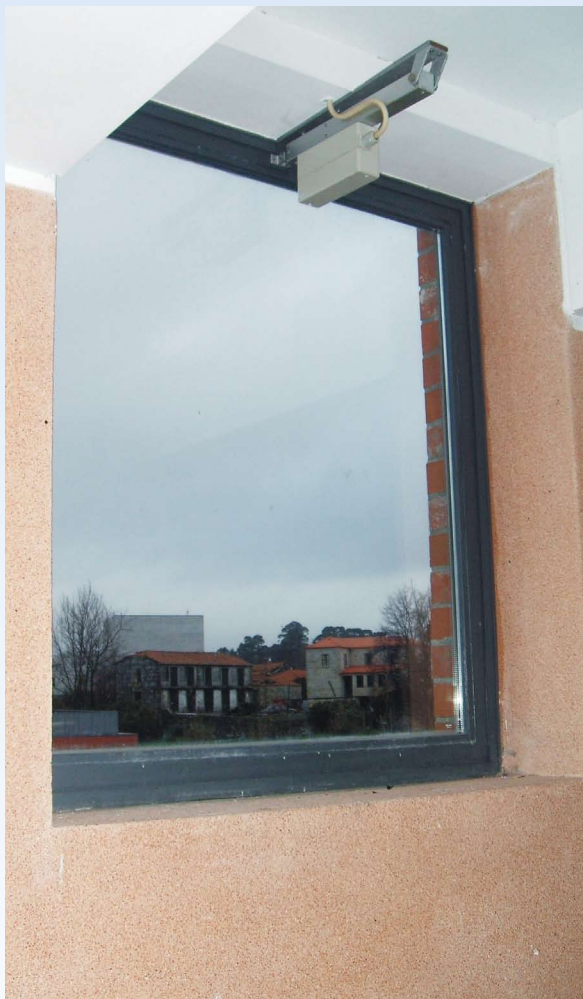
Figure 4. Openable window and operating mechanism.
