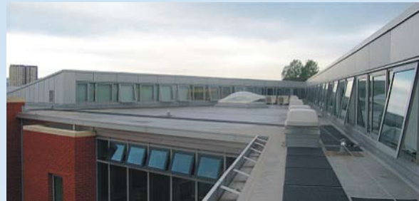
Figure 3. First floor roof showing clerestory opening lights.
