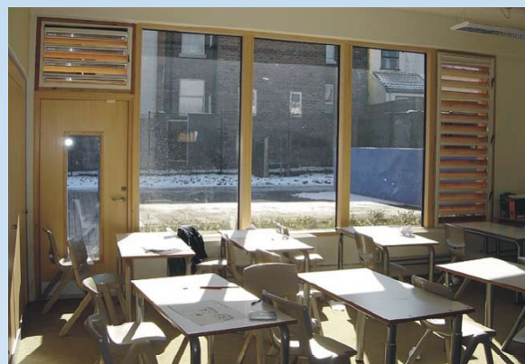
Naturally ventilated ground floor classroom
