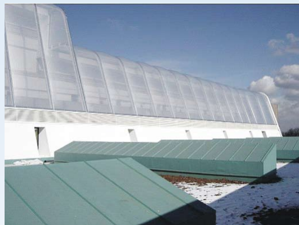
Figure 4. ETFE atrium and main hall roof.
