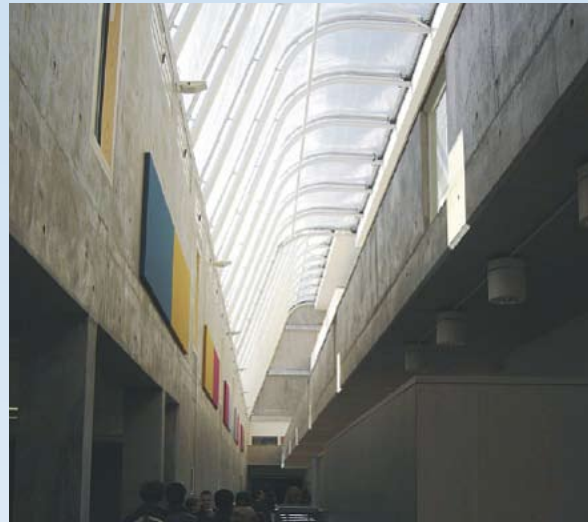
Figure 3. The atrium showing the ETFE translucent roof.
