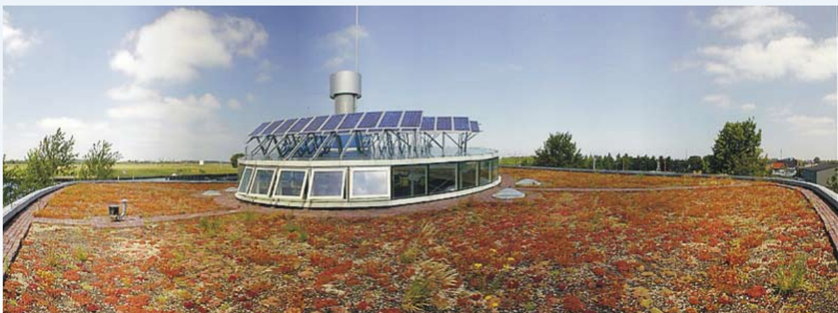
Figure 2. Roof of the building showing the 'chimney', atrium glazing and PV cells.
