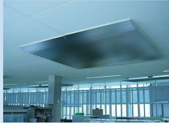
Figure 2. Open plan office showing reflecting surfaces.
