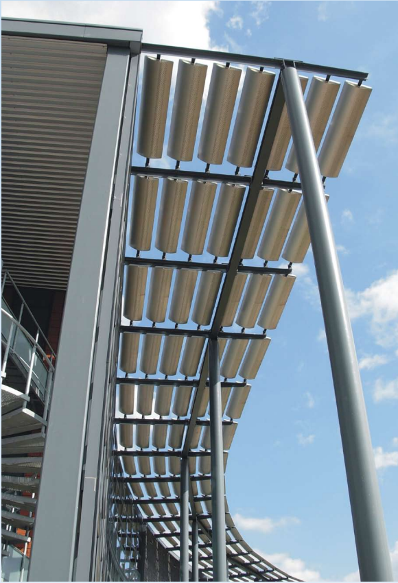
Figure 2. The brise-soleil incorporating PV cells.
