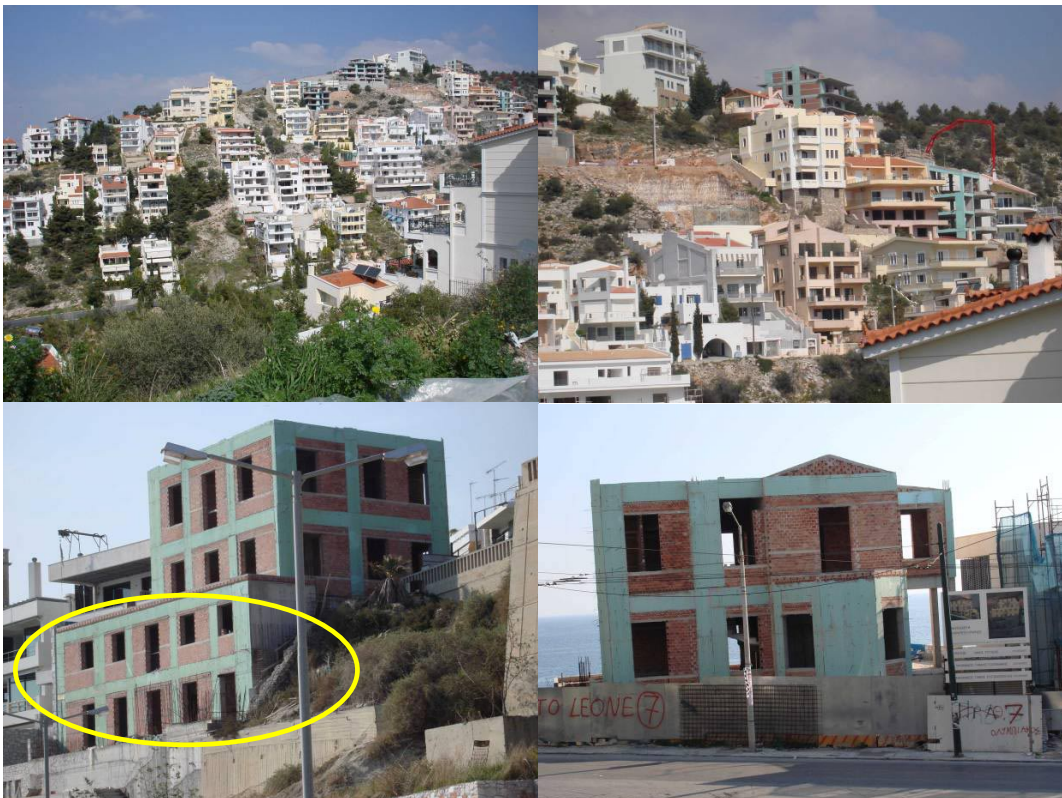
Fig. 4. IC cases exceeding the permissible floor spaces (basements in downhill not included in the surface permissible by the BC).
