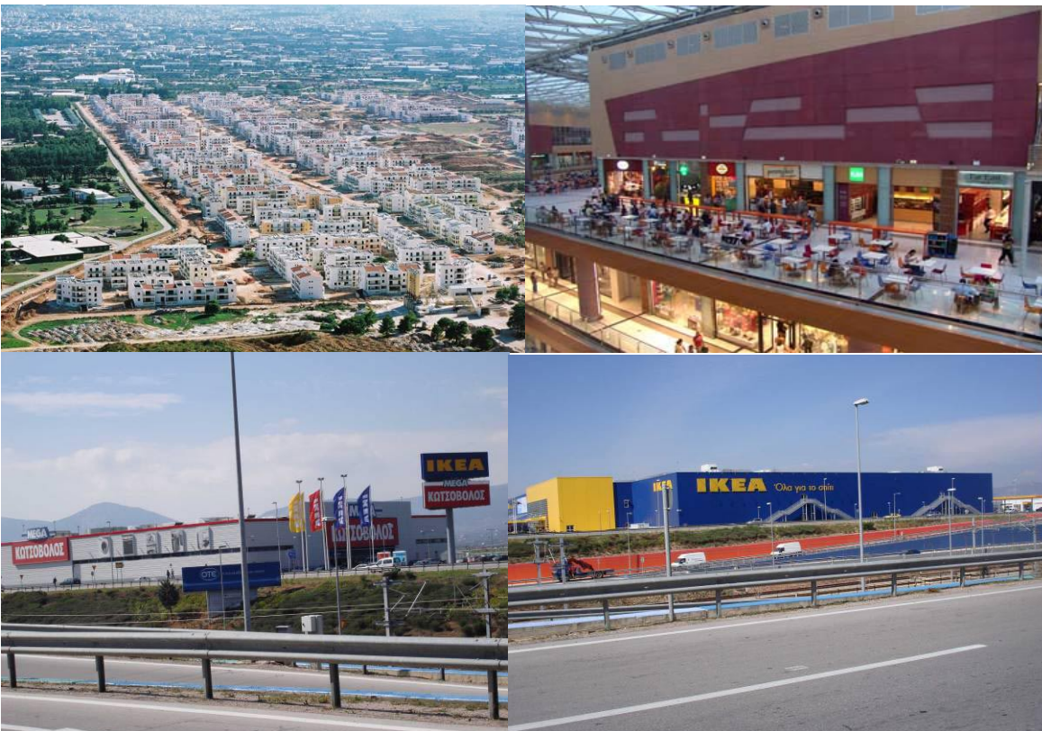
Fig. 10 Olympic Village, constructed not in accordance to zoning regulations and "the Mall", Department Store (1 st row) Commercial developments in the area of El.Venizelos national Airport (2 nd row)
