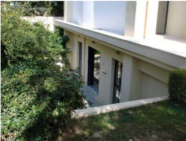
Fig.6 The basement of an office building turned into bureau.
