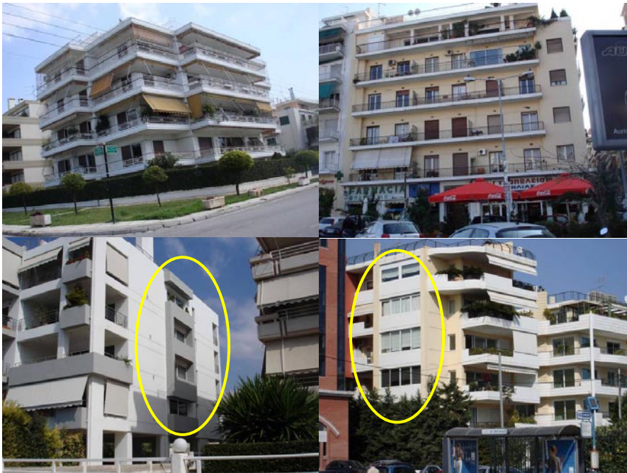
Fig.3 First row: Buildings without semi-open air spaces, and second row: buildings with informally closed semi-open spaces
