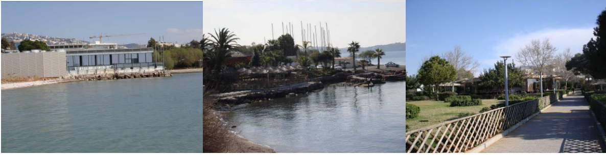
Fig.13 Illegal constructions in rent public land/ buildings located in privileged areas.
