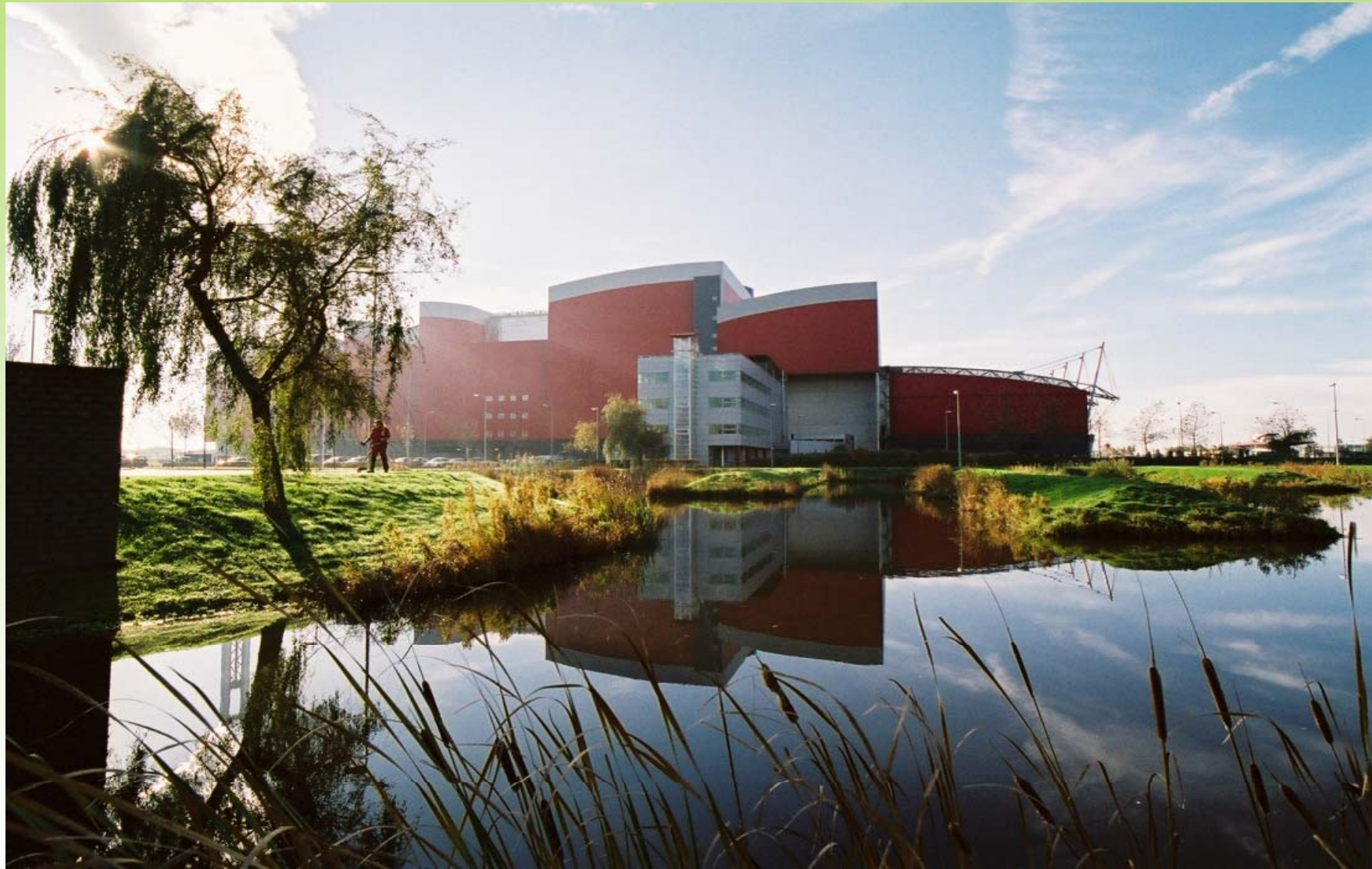
Alkmaar WTE, Netherlands
