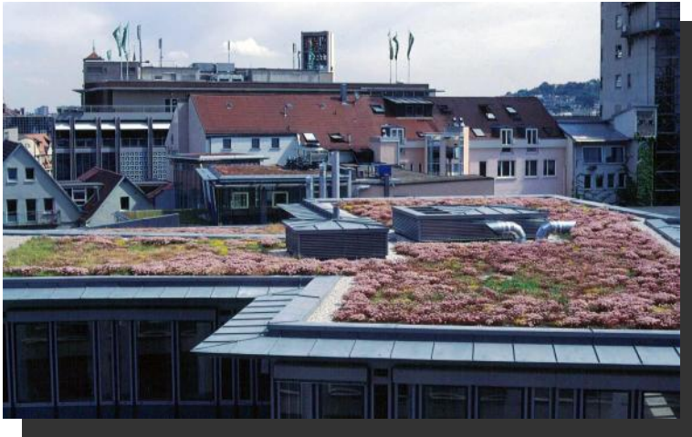
Extensive Green Roof - Low maintenance Green Roof
