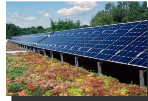
Green Roofs and Photovoltaics
