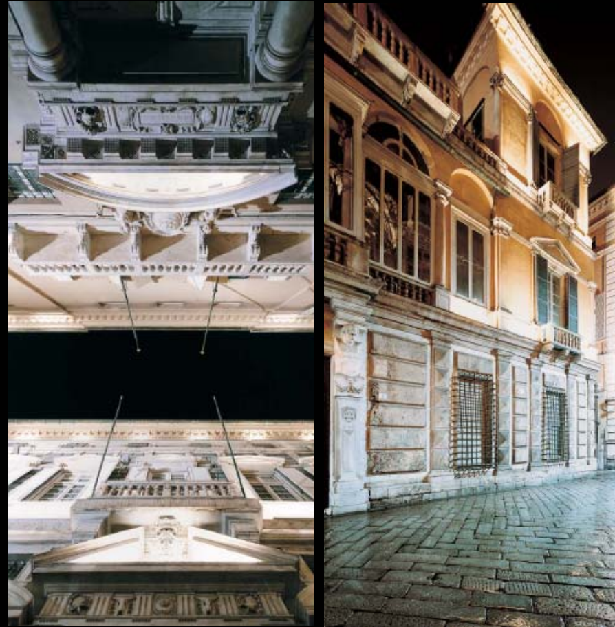
Via Garibaldi, Genova, Italy, ARTEMIDE Architectural
