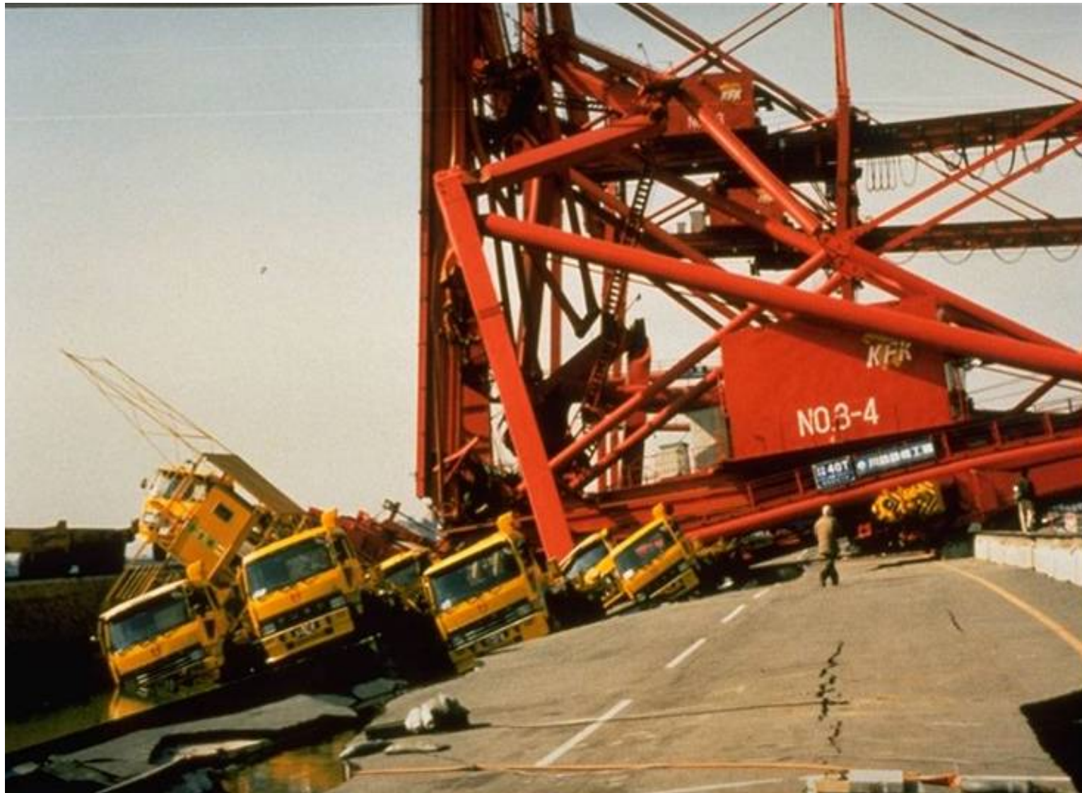
Collapse of crane due to lateral movement (~2 m) of quay wall on Rokko Island. Note settlement of 1-2 m also occurred behind wall.
