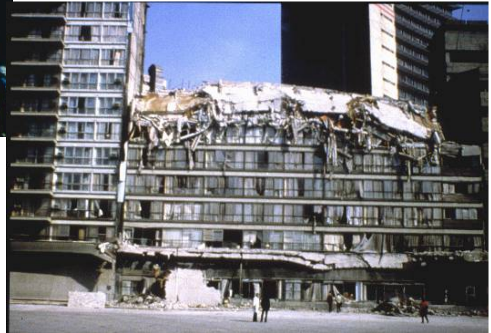
Failure of Top Floors, Hotel Continental
